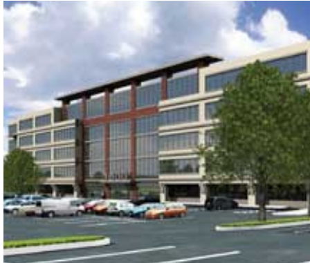
Picture 4: Office Building 1,000 Continental, King of Prussia, PA with EnOcean enabled wireless sensors
